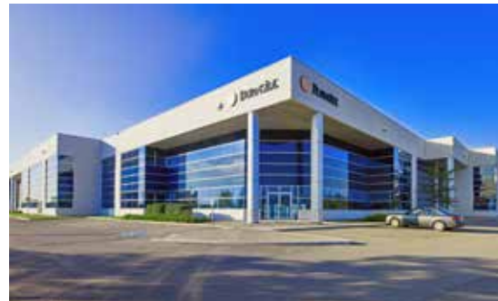
Industrial Building: 6990 Creditview Road , Mississauga, owned by MNBP Single & Flex Holdings Inc. and managed by QuadReal Property Group.
